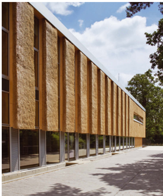
↓ FIGURE 1: UEA's award-winning Enterprise Centre meets both Passivhaus and BREEAM 'Outstanding' standards
